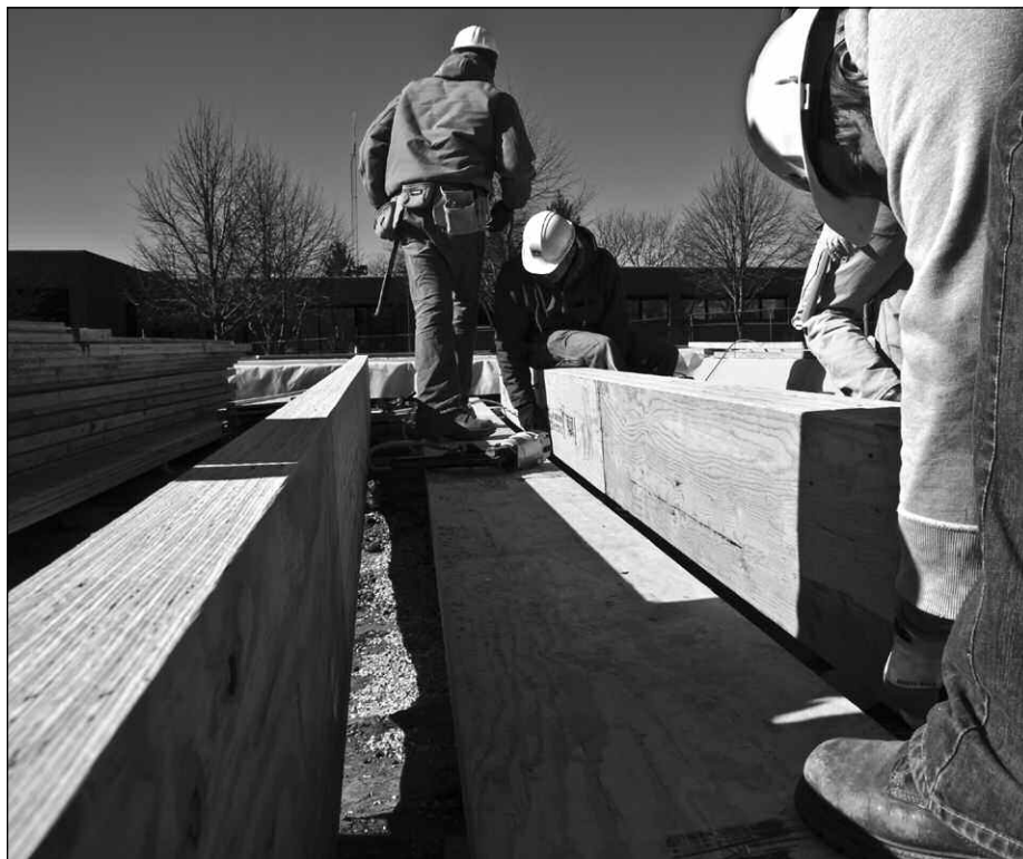
LVL beams used in floor framing.
